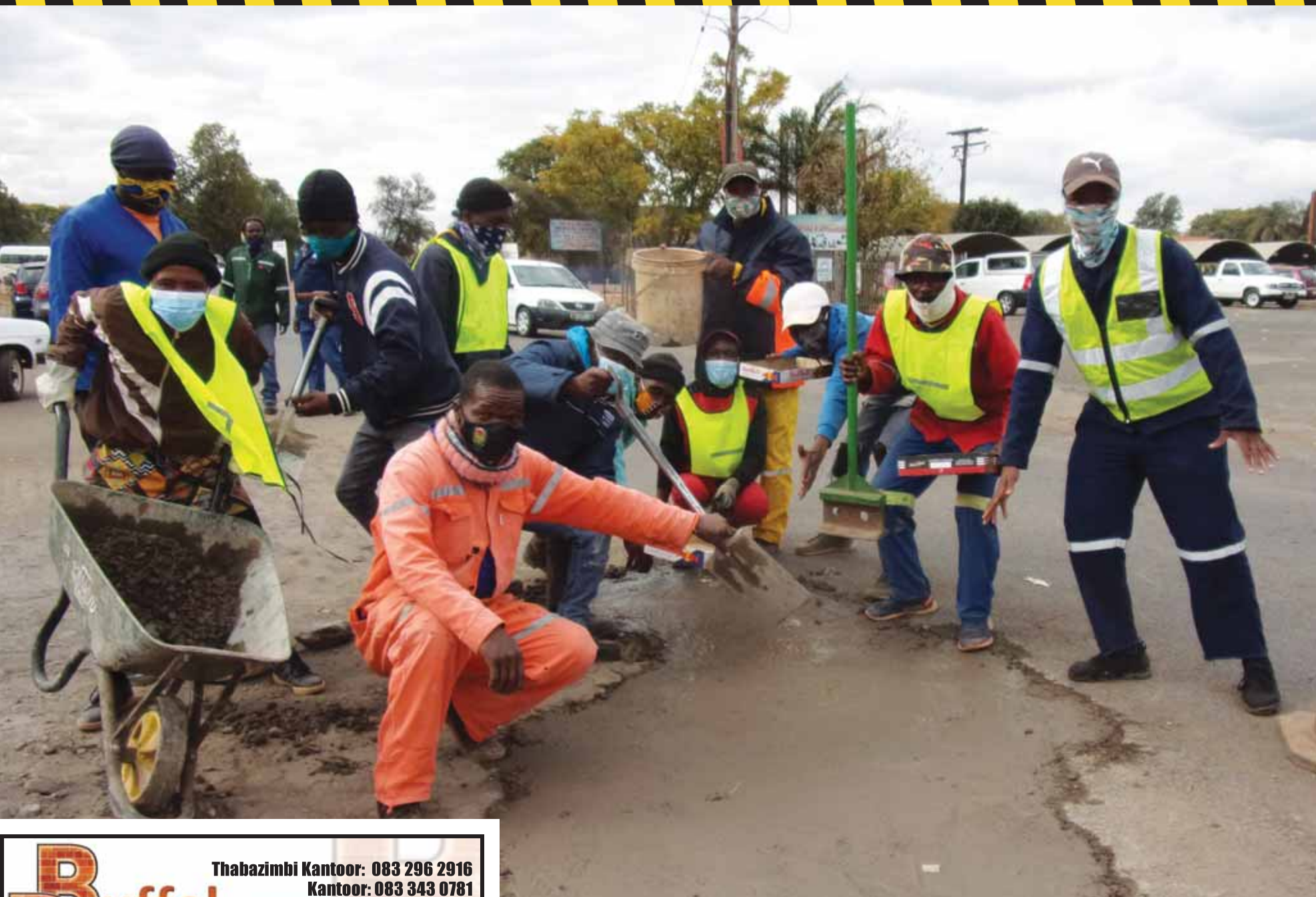
Northam community members took to the streets to repair potholes.
